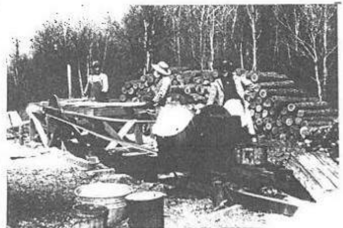
Lathe and shingle mill used in constructing Salem. Left to right: Sievert Berkness, Tillie Beck and Carrie Berkness.
